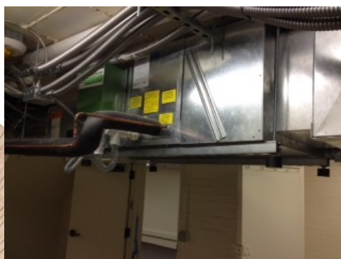
All of the Unico Green Series units Top: Plenum configured in "H" style pattern
