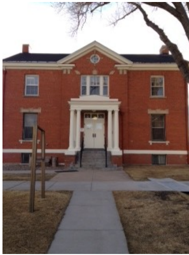
The front of the building
