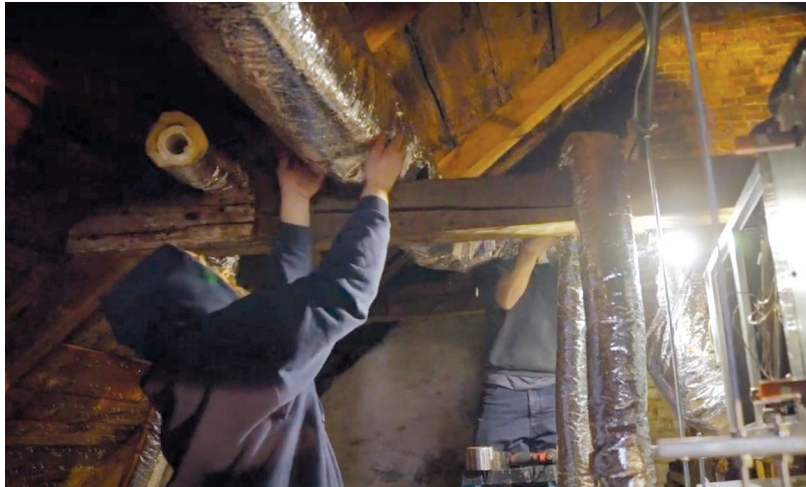
Installers situate the compact Unico System main duct.
