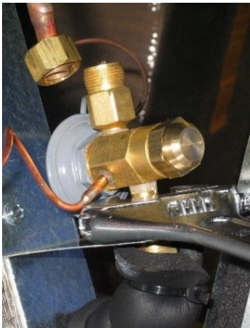
Figure 9. Attaching TXV to Distributor
