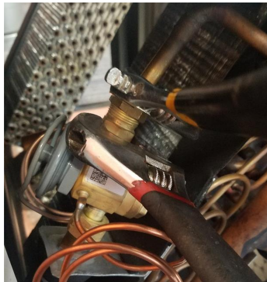
Figure 10. Attaching TXV to Liquid Line
