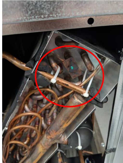
Figure 24. Cut zip ties before installing TXV
