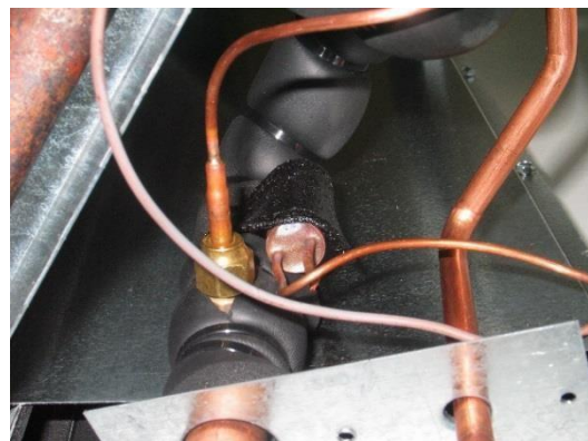
Figure 30. Bulb Secure Clamp and Cork Tape
