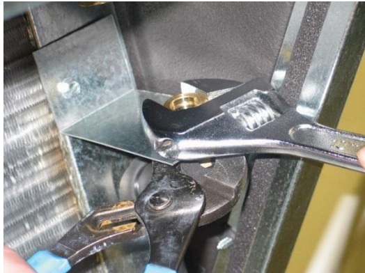
Figure 23. Remove Nut
