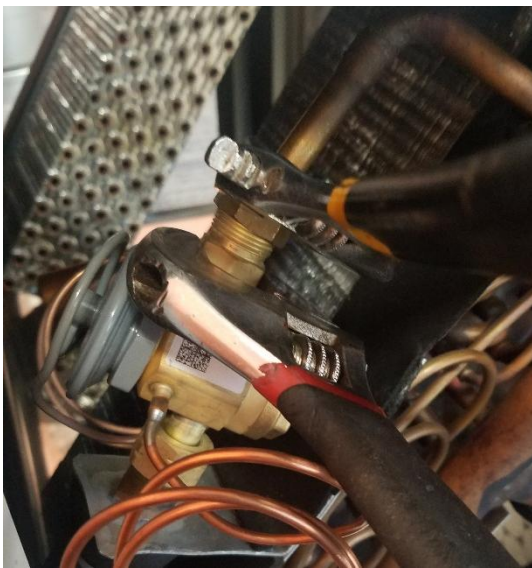
Figure 10. Attaching TXV to Liquid Line
