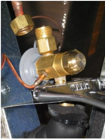
Figure 9. Attaching TXV to Distributor
