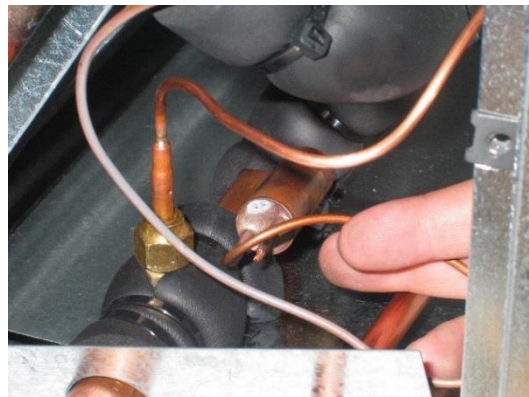
Figure 29. Thermal Measuring Bulb Placed on Copper Tube.
