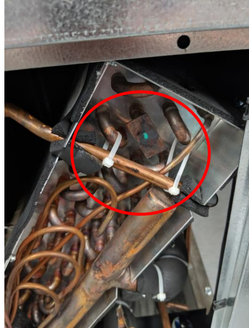
Figure 24. Cut zip ties before installing TXV
