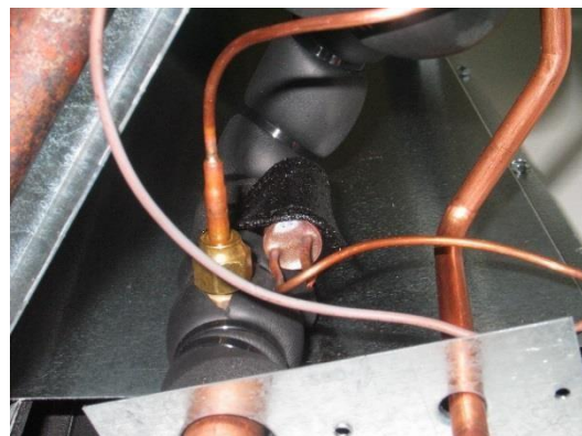
Figure 30. Bulb Secure Clamp and Cork Tape
