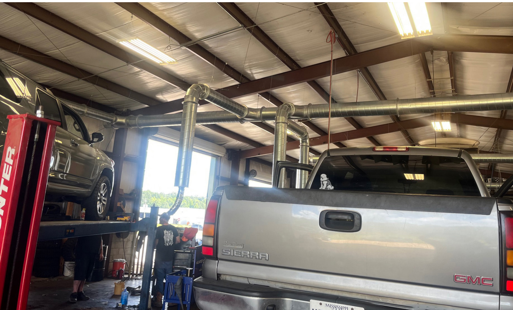
Unico Spot Cooling uses flexible tubing to deliver cool air to the mechanics at their workstations rather than inefficiently trying to condition the entire space.
